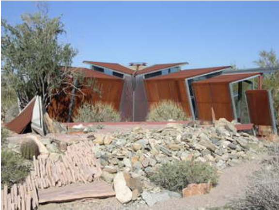
USA: Steel (rusted) and structural glass.
